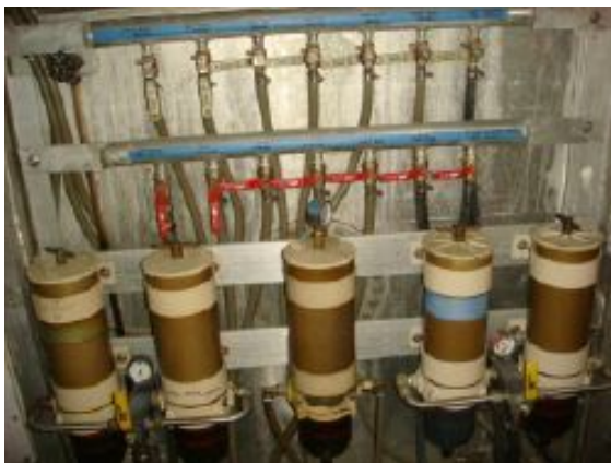
> 60' Custom Trawler fuel manifold
