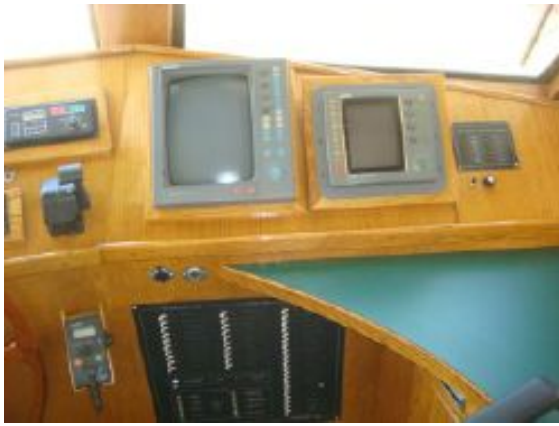
> 60' Custom Trawler pilothouse helm starboard
