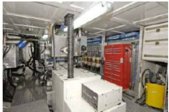
> 60' Custom Trawler engine room aft
