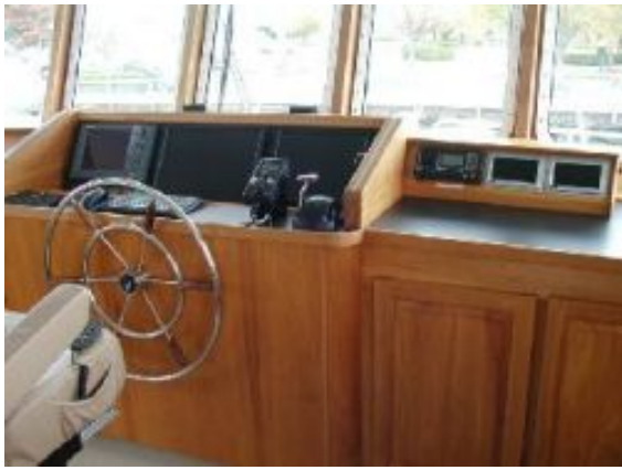
Pilotage Console, Radio and CCTV Monitors
