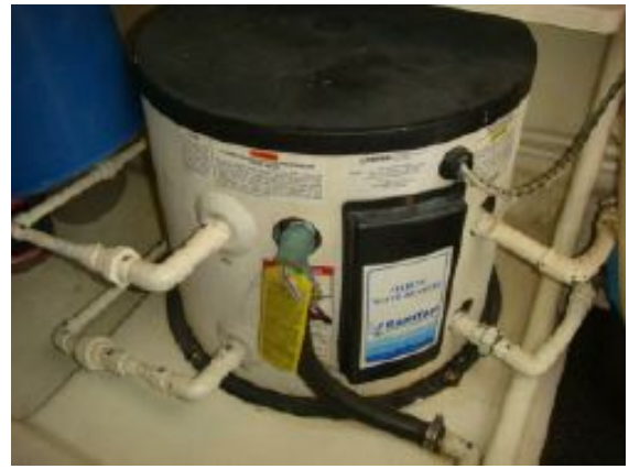
> 50' Alwoplast port water heater
