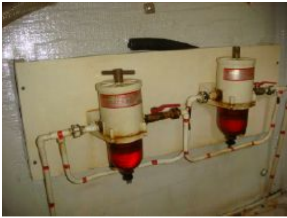
> 50' Alwoplast starboard Racor fuel filters
