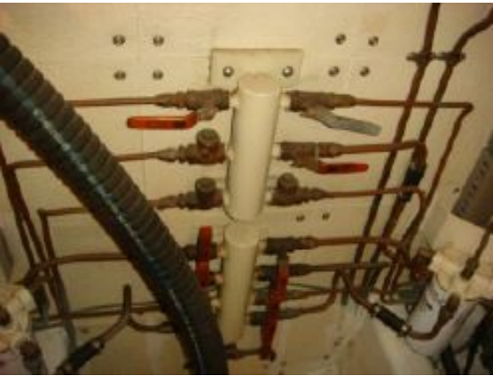
> 48' DeFever fuel manifold
