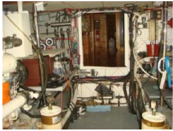
> 47' Tradewinds engine room forward
